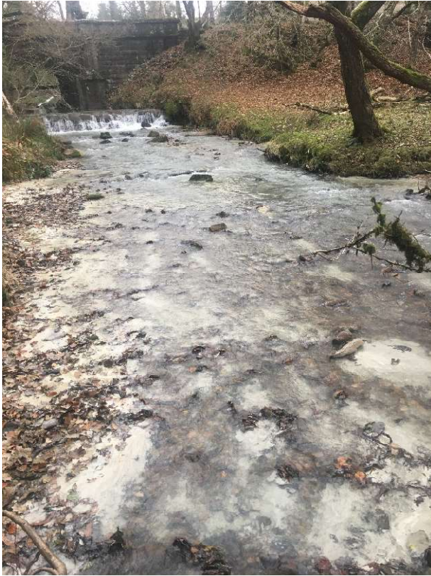
Figure 21: Deposits remaining below Piall Bridge recorded by Tony Hawkins 0950h 14Dec22
