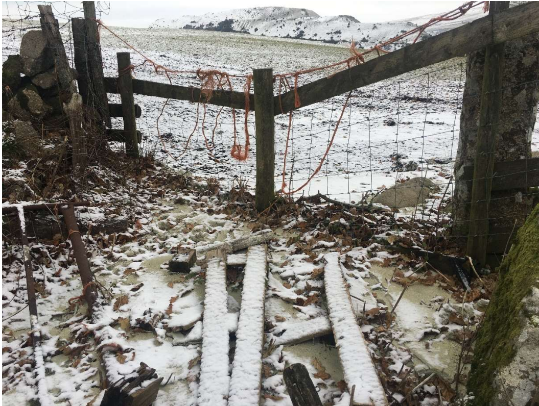
Figure 23: Recent deposits of kaolin-like material evidencing overland pollution running into the top of Broomage Wood from field above Tin Park recorded by Tony Hawkins 1020h 14Dec22
